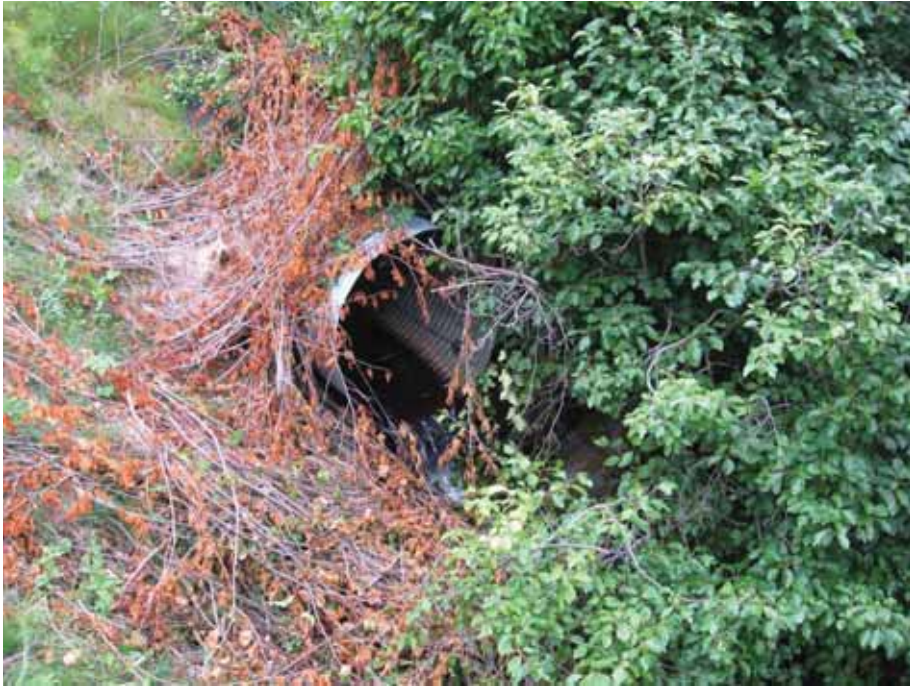
“Bear” Creek highway culvert outlet
