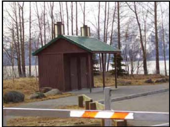
Photograph 17 – Chugach State Park – Indian Creek. Pit toilets.
