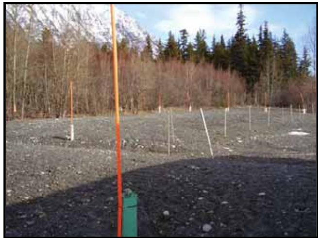
Photograph 8 – Essential Gas Station leach field constructed in 2005.
