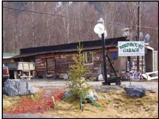
Photograph 31 – Additional view of the Birdhouse Garage.
