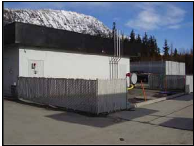
Photograph 1 – Essential Gas Station gasoline UST area.
