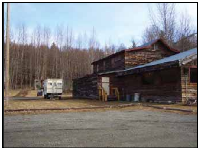
Photograph 15 – Rear of Indian Valley restaurant.
