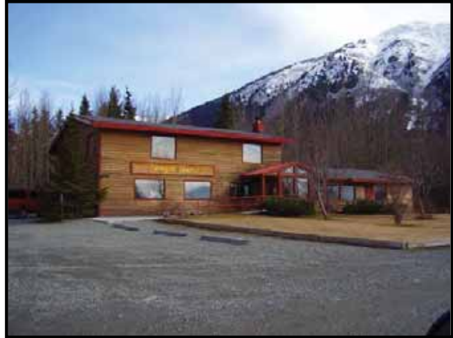
Photograph 16 – Turnagain House restaurant located at approximately MP 103.
