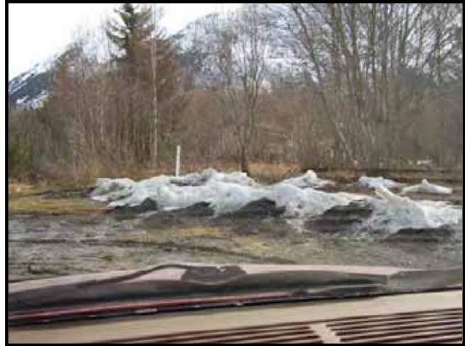
Photograph 28 – Bird Ridge Café septic system located approximately 50 feet north of the Seward Highway.
